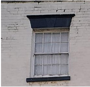
Figure 26 8/8 pane sash window, 32 Lower HS
