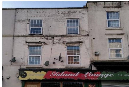
Figure 22 Rendered and painted brickwork typical of 19th century frontages
