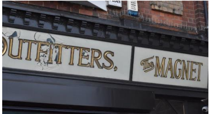
Figure 56 Former Outfitters, 13 Market Place
