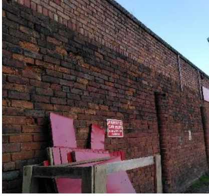
Figure 23 Wall, North of Shambles Car Park
