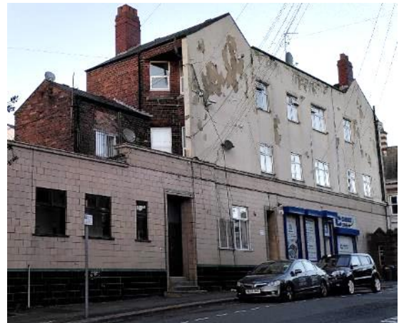
Figure 18 Former George Inn, side elevation viewed from The Shambles.
