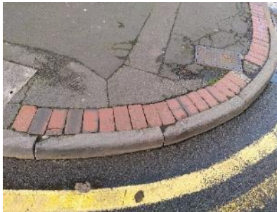
Figure 73 Paving Russell Street
