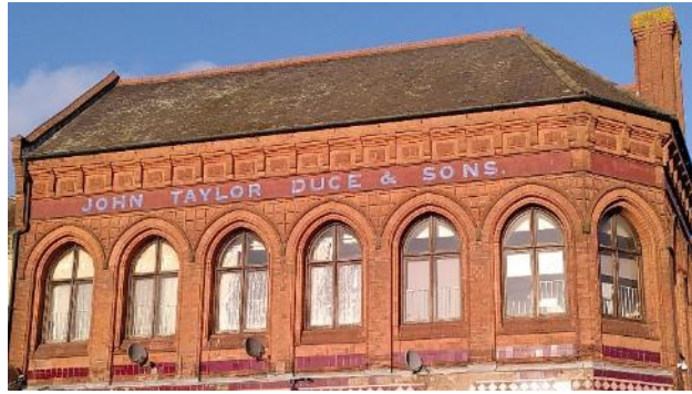
Figure 54 Duce & Sons Brewers, 27 Market Place
