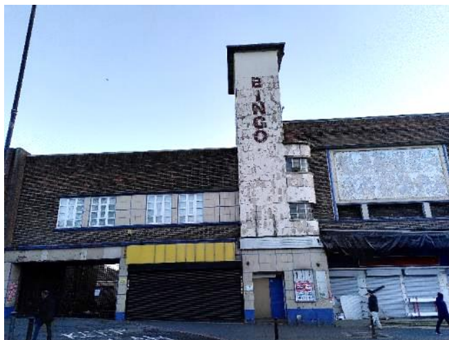
Figure 87 Former Cinema, Walsall Street.
