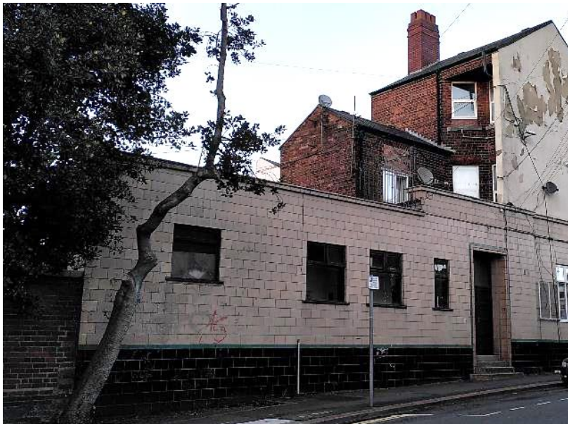
Figure 78 Former Public Conveniences, The Shambles
