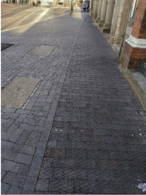
Figure 67 Blue diamond paving, Market Place
