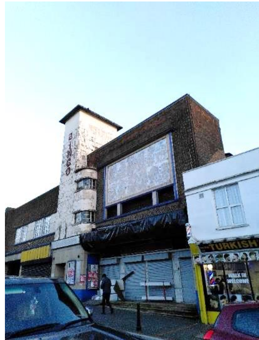
Figure 69 Locally listed former Gaumont Cinema, Walsall Street.
