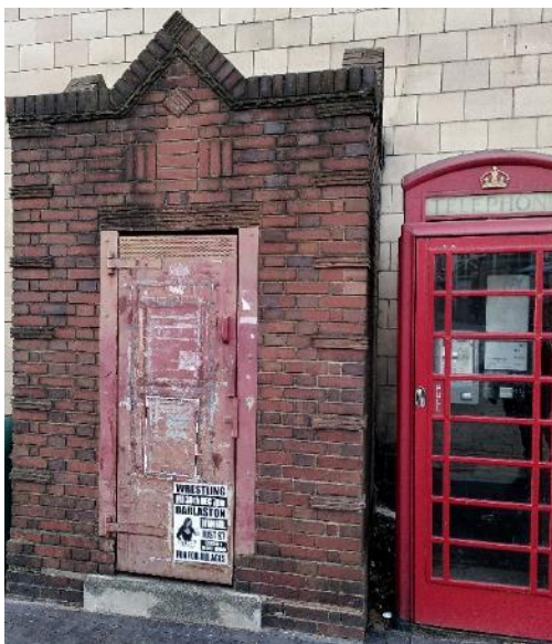
Figure 63 Police Box, Shambles.
